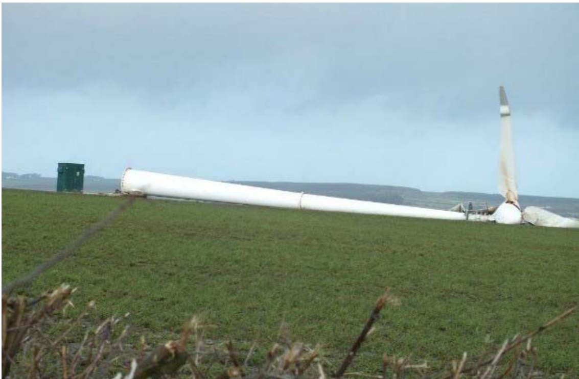
Figure 3 Image from a press report in September 2014 3 showing a toppled turbine
