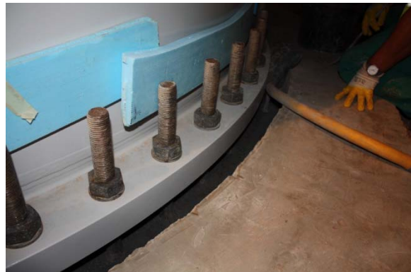
Figure 21 Under-base grouting on a large wind turbine
